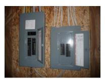
*Main Power Panel Size:* 200 amp - The ampacity of the main power panel appears to be adequate for the structure as presently.
