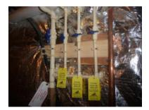
*Interior Supply Piping Size:* The interior water supply piping is 3/4" in diameter. It then reduces to 1/2" or 3/8" risers.
