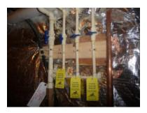
*Functional Supply:* Satisfactory: By testing multiple fixtures at one time, functional flow of the water supply was verified.
