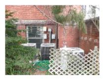
AC unit #4 was in 1988, this system cools the second floor, the thermostat is located on the second level. This system was operational. However, it has passed its useful life and you should budget to replace it. There was a repaired leak under the air handler in the ceiling of the front left second floor landing. The air handler is located in the attic space above this landing. When replacing the system, you should consider installing the air handler and compressor in a more convenient location
